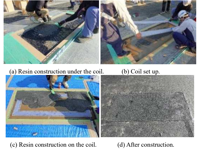
Fig. 9. Case coil construction procedure.
